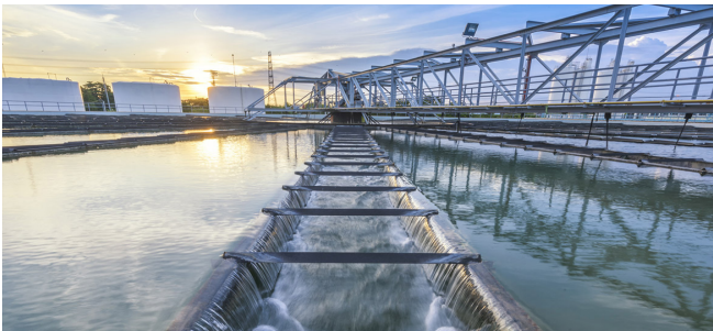
WATER TREATMENT PLANT, UK
