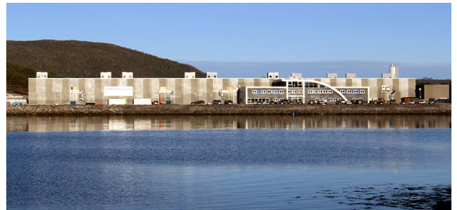
SEWAGE TREATMENT PLANT, SWEDEN
